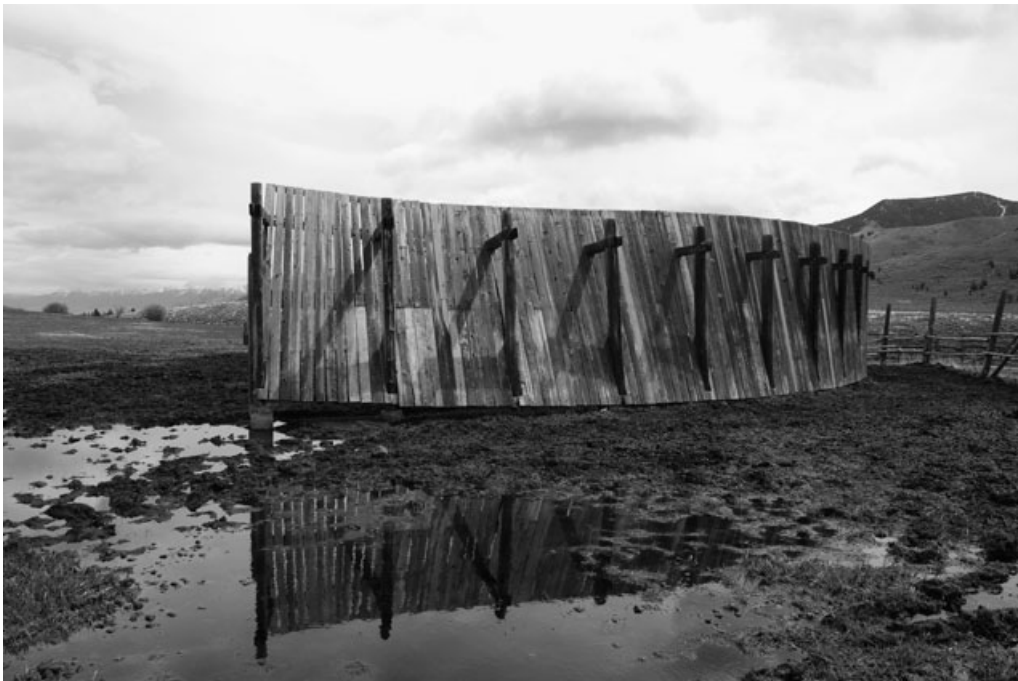
9. B Bar Wind Shelter , built Summer 2000 on the sustainably operated B Bar Ranch where the lumber was harvested and milled. The straightforward detailing allows repair over time as elements and horses inflict wear. Southwest of Emigrant, Montana June 3, 2010. (Photo by Chris Taylor.)
