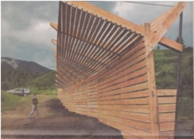
Steve Warming looks over a horse shelter on a ranch south of Livingston Tuesday. Warming is part of a team of Montana State University architecture students that designed and built the structure.
